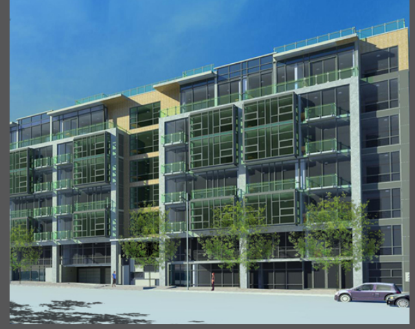
residential units on Illinois Street
